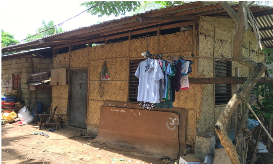
Figure 1. The house of one of my informants in New Princesa with concrete flooring and local coconut fibers used for the walls. Corrugated steel is commonly used for roofing.
